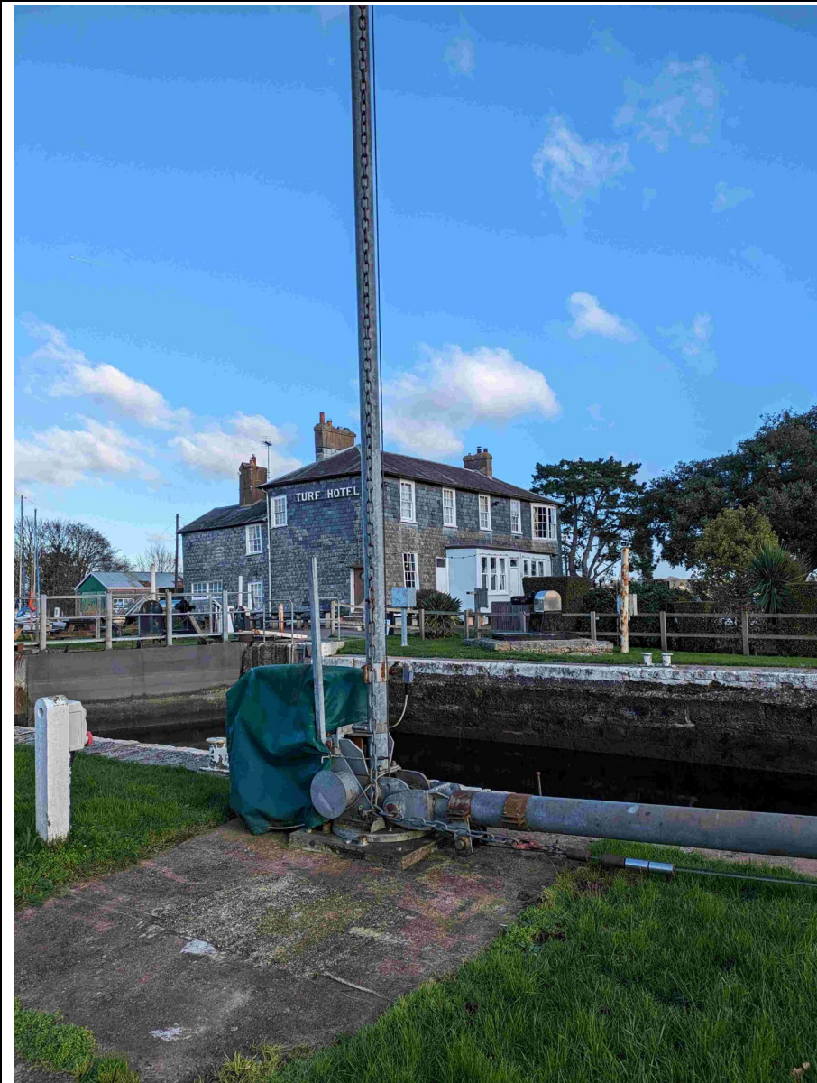
Image B19. Turf Lock Masting Derrick
