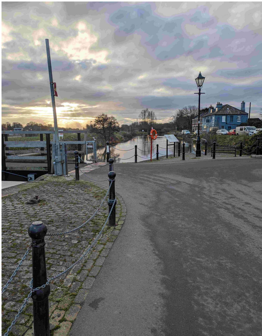
Image B13. Example Canal Bridge edge protection LSE and Signage
